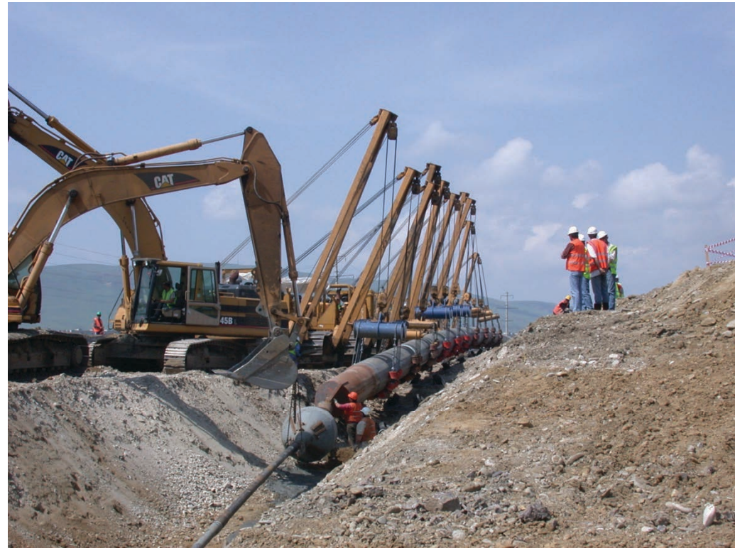
Pullback operations for a 48-inch pipeline in the Republic of Georgia.
