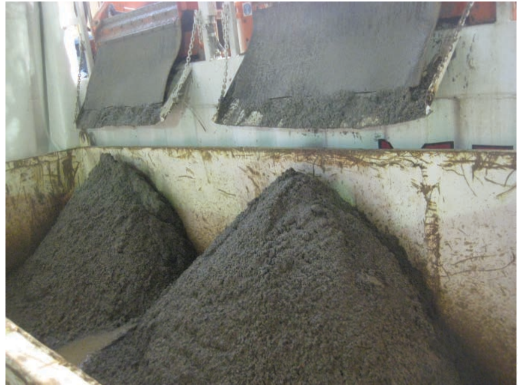
Cuttings generated from a sandy soil HDD installation.
